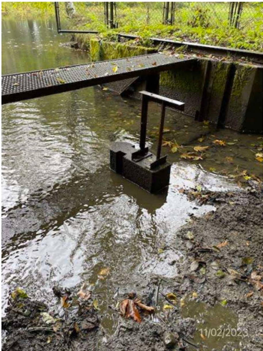
Nov 2 nd 2023, Boards removed, low water levels not flowing from lake
